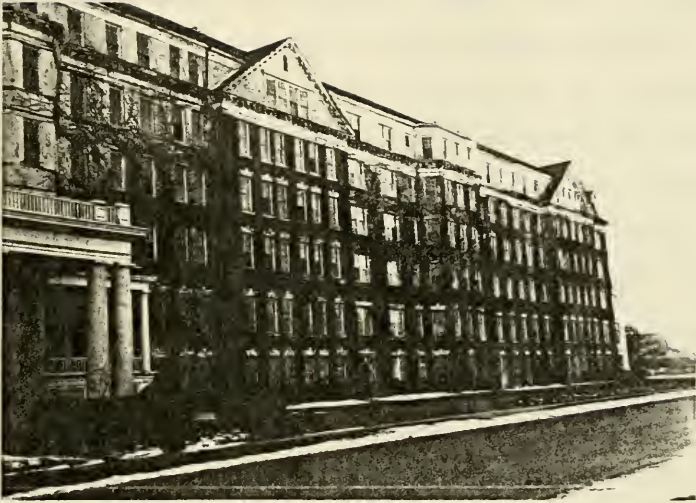
Plate 42: North Wing, North Elevation, 1985
